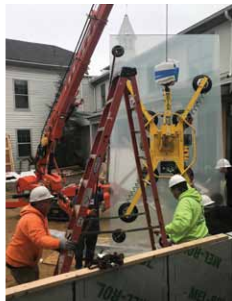
The installation of glass panels for the 12 ft-cube is underway as part of the current round of renovations.
